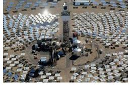
A power tower produces electricity from sunlight by focusing thousands of sun-tracking mirrors, called heliostats, on a single receiver sitting on top of a tower. The receiver captures the thermal energy of the sun and stores it in tanks of molten salt (to the right of the tower) at temperatures greater than 500 degrees centigrade.
